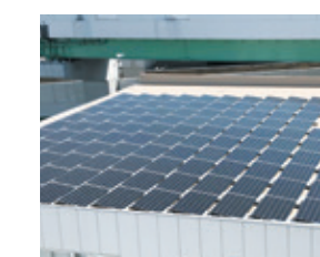
Rooftop of the head office
