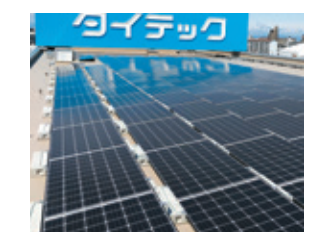
Rooftop of the head office factory
