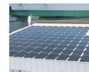
Rooftop of the head office
