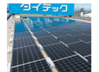
Rooftop of the head office factory
