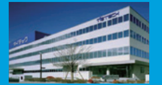
TECHNO HORIZON CO., LTD. • Head Office Factory • Nagoya Office
